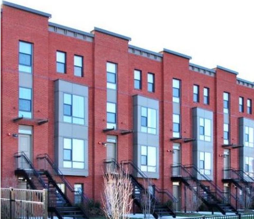
The SeVerna Phase I, Northwest One
